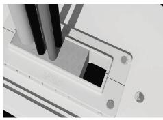
9. Fill remaing space with unprepared modules.
