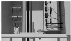
11-12. Tighten the PTG 40 wedge until it is almost even with the frame surface to obtain IP 65/67 rating.
