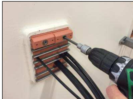
Tighten the two bolts evenly in steps.
