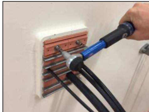
Or use a torque wrench. Maximum torque is 20 Nm.
